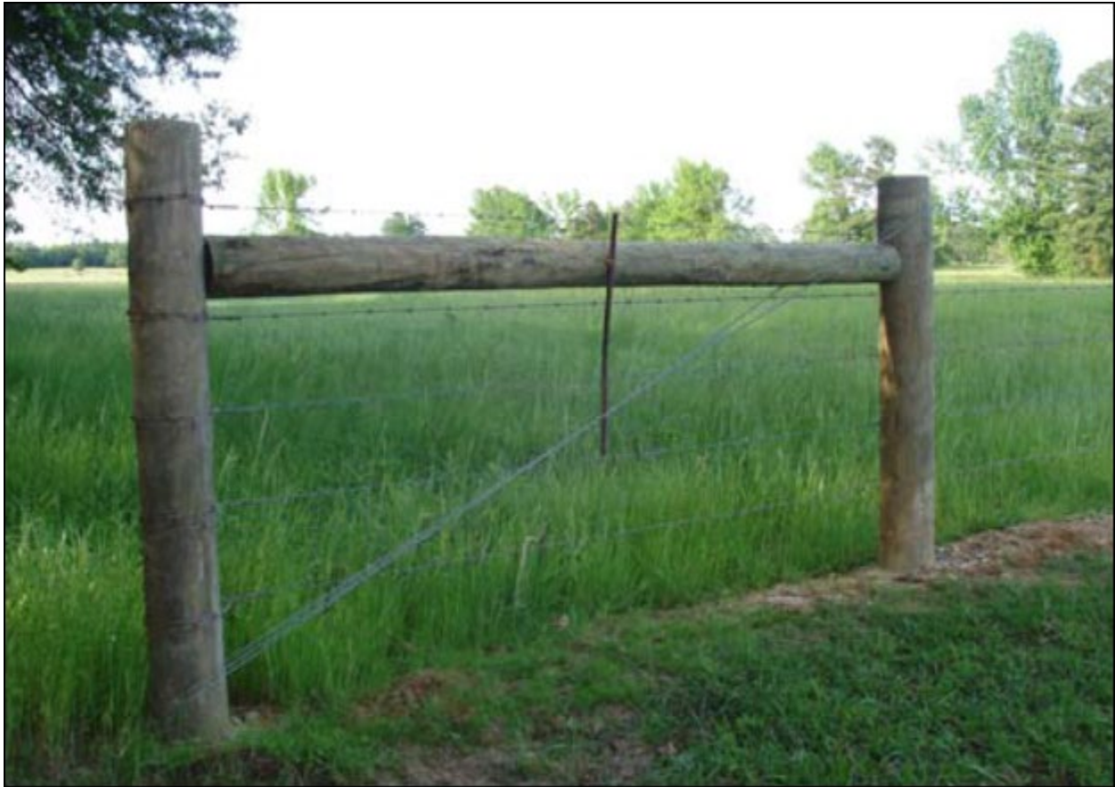
Common barbed wire fence H-brace
